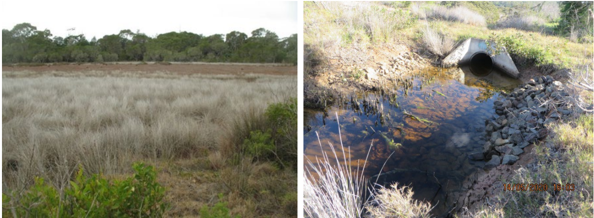
Figure 6-3 Saltmarsh habitat east of south runway (left) and 300mm culvert under Southern Access Track.
